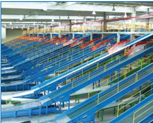
Distribution/ Parcel Service
